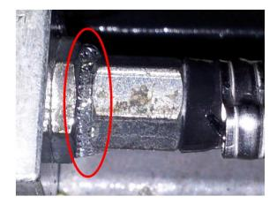
Within the red marking, foam formation can be seen at the gas pipe. This is an indication of leakage.
